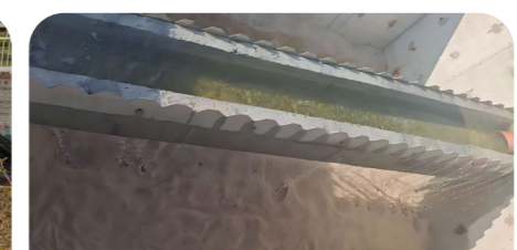
Dredge the reclaimed water reuse pipeline
